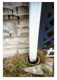
to carry sewage in a separate set of pipes from stormwater. It is illegal for rainspouts (or any stormwater drain) to be connected to a separate
